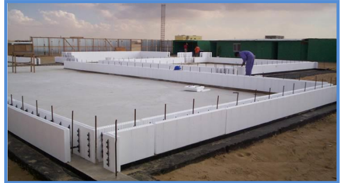
STEP 2/ Install ICF Blocks
